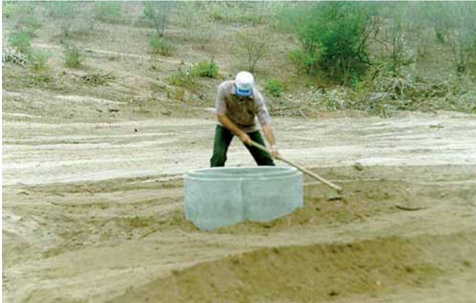
Photo 12 –Underground Dam Completion Stages
