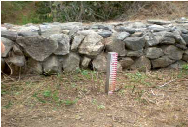
Photo 6 - Stone Dam – Zero Base Technology (TBZs)
