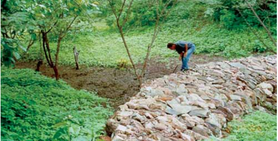
Photo 7 – Effect of Sediment Retention and Resurgence of Herbaceous and Arborous Vegetation after Winter Period.
