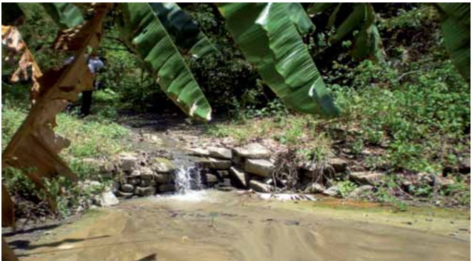
Photo 8 – Effect of Sediment Retention and Resurgence of Herbaceous and Arborous Vegetation after Winter Period.
