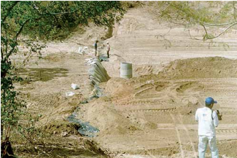
Photo 11 –Underground Dam Completion Stages Source: João Bosco de Oliveira.
